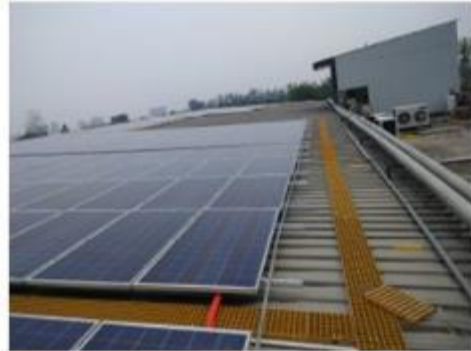
Roof top solar supplier site, Gurgaon
